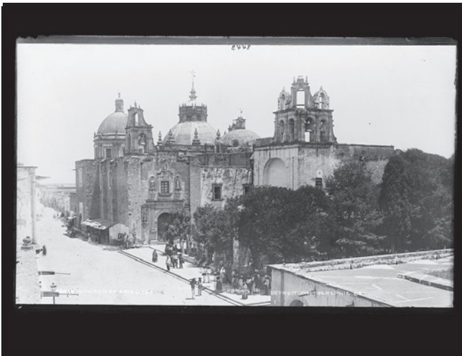
San Diego Church, Aguascalientes, Mexico.
